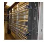
Spring return actuators are also known as fail-safe actuators because they return the damper to an open or closed position that is safe for the environment where the damper is located.
